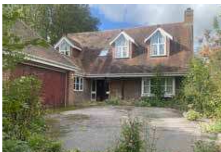
After an initial letting, the New Vicarage in School Road has remained empty
