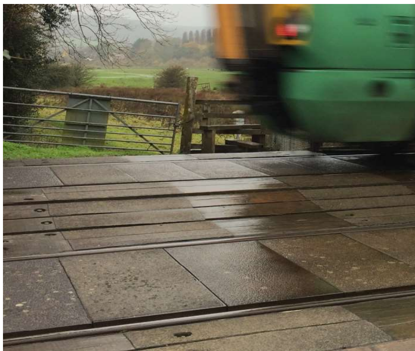
An accident waiting to happen: the dangerously slippery crossing surface
