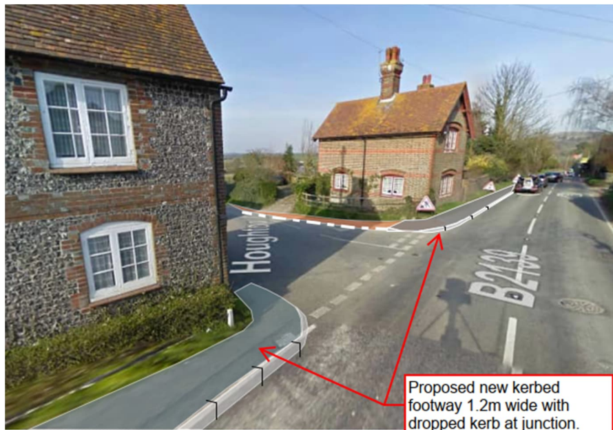
Figure 7 – Photomontage showing the proposed footway at the junction with Houghton Lane and the B2139
