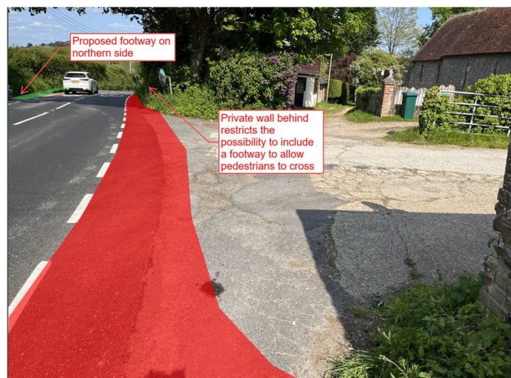
Figure 15 – Proposed footway across Houghton Farm Access
