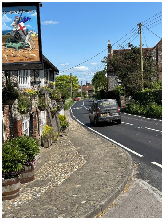
Figure 3 – Section of footway outside the George and Dragon Public House
