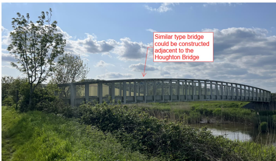
Figure 19 – Existing pedestrian footbridge
